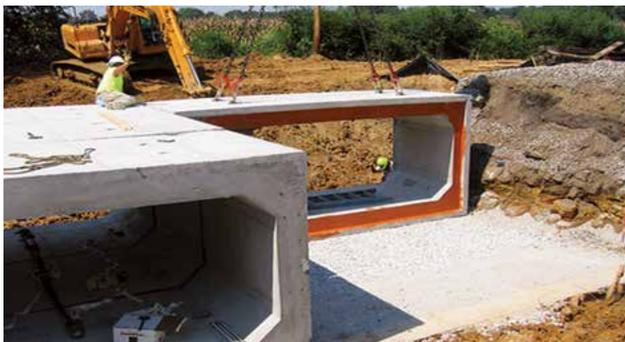
Fig. 14 Bedding Below Precast Concrete Segmental Box Cell
