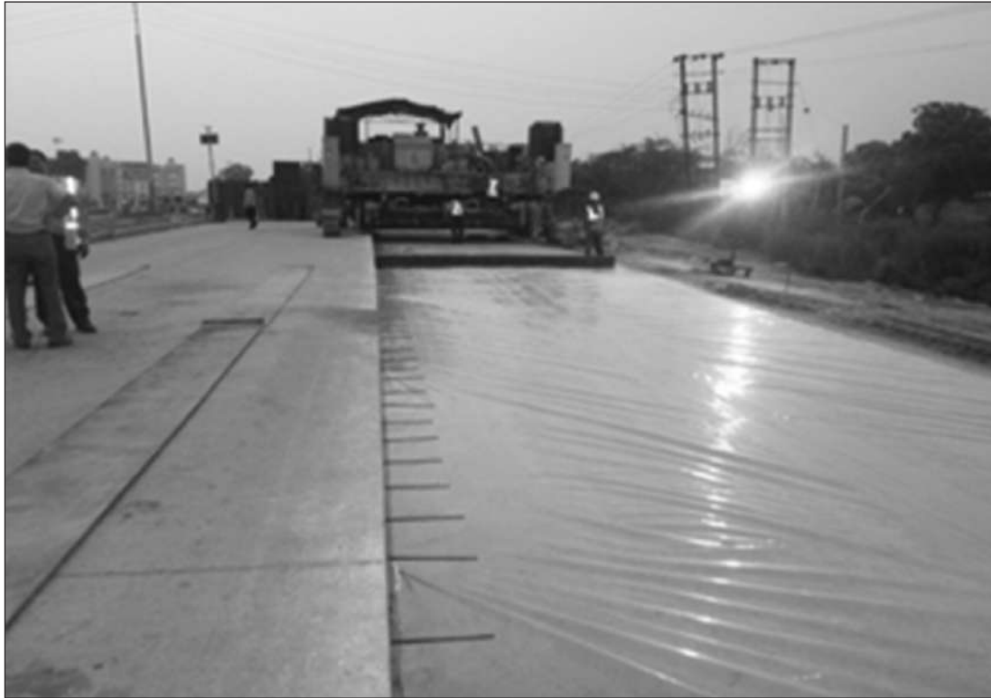
Tie Bars Installed at Longitudinal Joint
