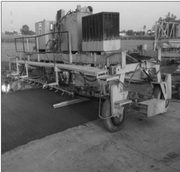
Laying of PQC for Widening
