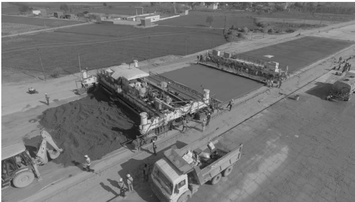
Fig. 16. A View of Slip Form Paving Train
