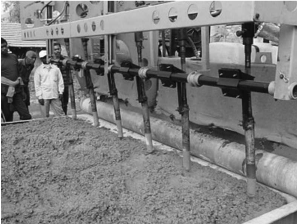
Fig. 17 Fixed Form Paver with Vibrators and Roller
