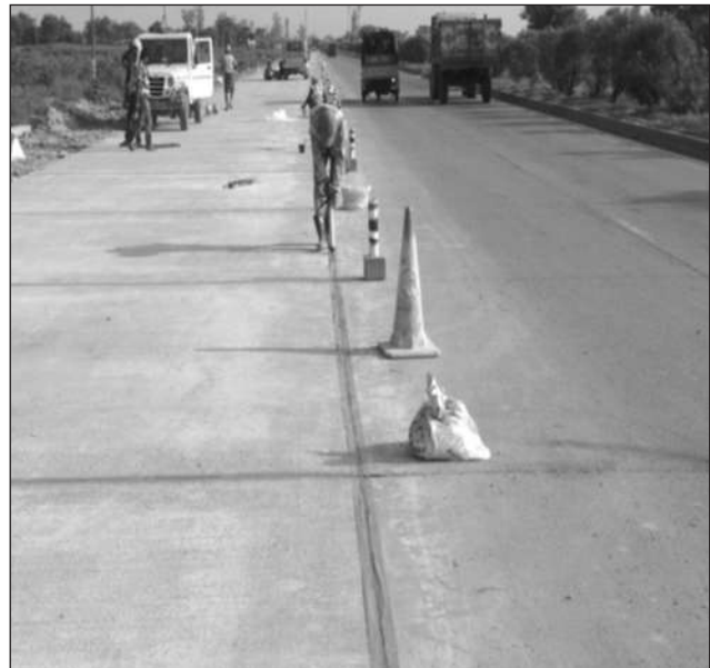
Transverse Joints of Old and New PQC Aligned in Line
