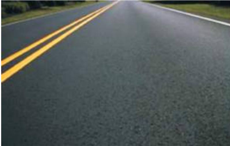
Photo 7.2.2 A View of Smooth Surface
