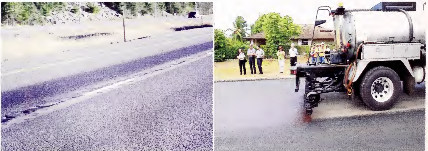
Photos 5.5 & 5.6 Fog Seal in Progress on a Oxidized Surface
