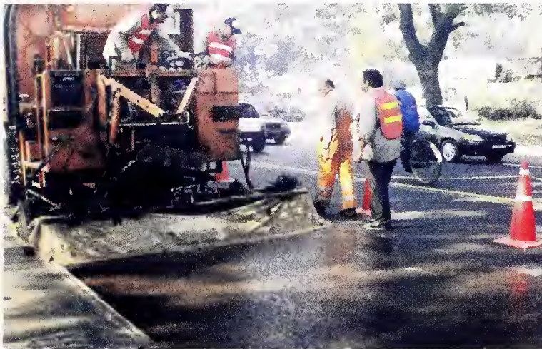
Photo 11.6 Microsurfacing in Progress and Microsurfacing Process
