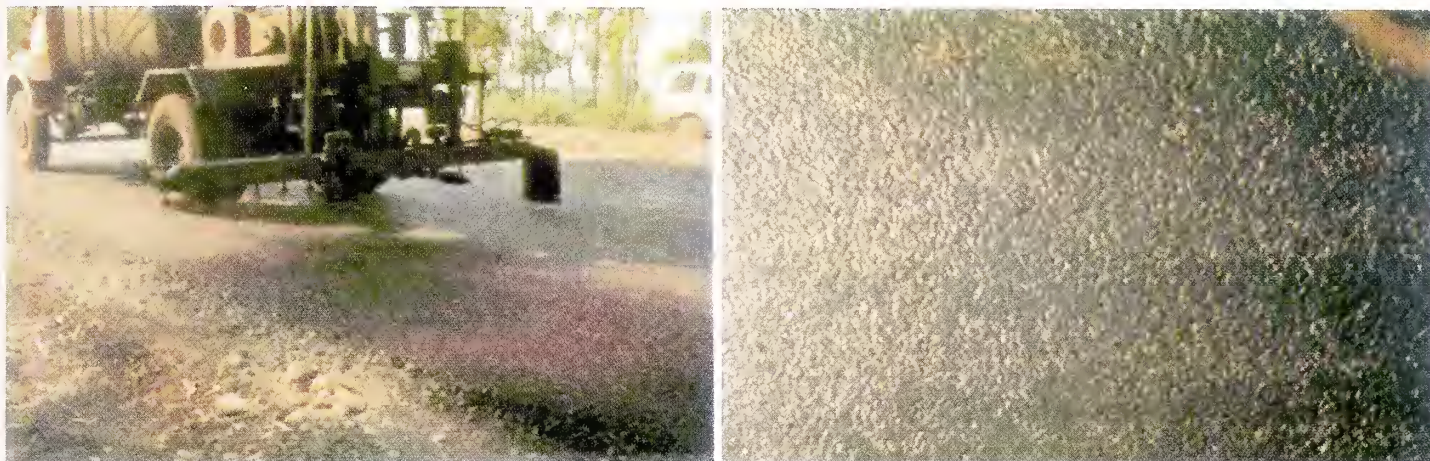
Photos 5.1 and 5.2 Priming in Progress Using Bitumen Emulsion
