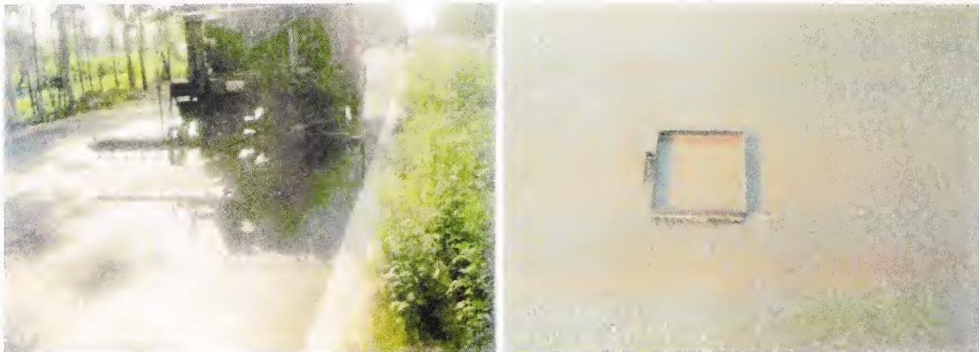
Photos 5.3 & 5.4 Application of Tack Coat Using Bitumen Emulsion and View of Good Tack Coat
