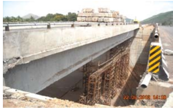
Photo 8 Load Testing by Static Method
