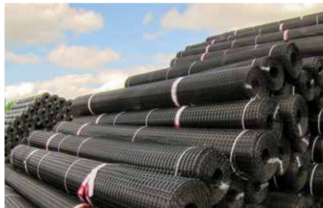
Fig. 6.3b Geogrid Rolls at Site
