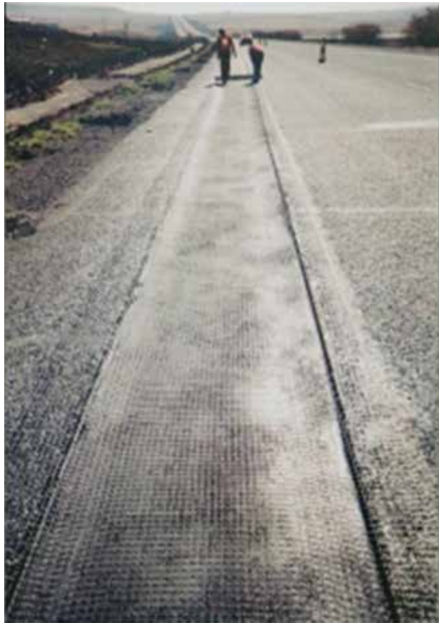
Fig. 5.11 Glass Fibre Grid placed on Levelling Layer Prior Paving
