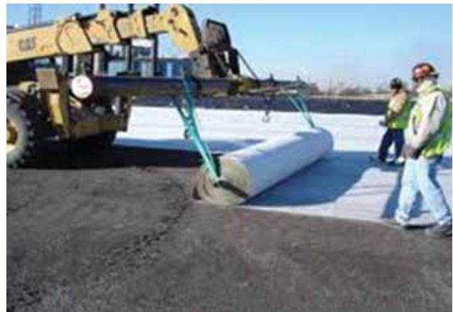
Fig. 6.2 Unrolling of Geosynthetic Roll
