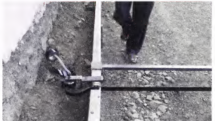
Fig. 5(m) Typical Tightening Device
