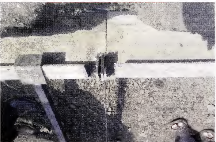
Fig. 5(n) Anchoring of Strip
