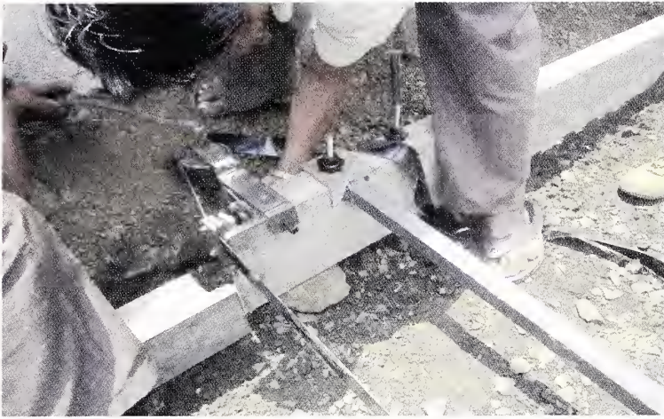
Fig. 5(j) A Close up View of Fixture of HDPE Separation Strip and Spacer Bar
