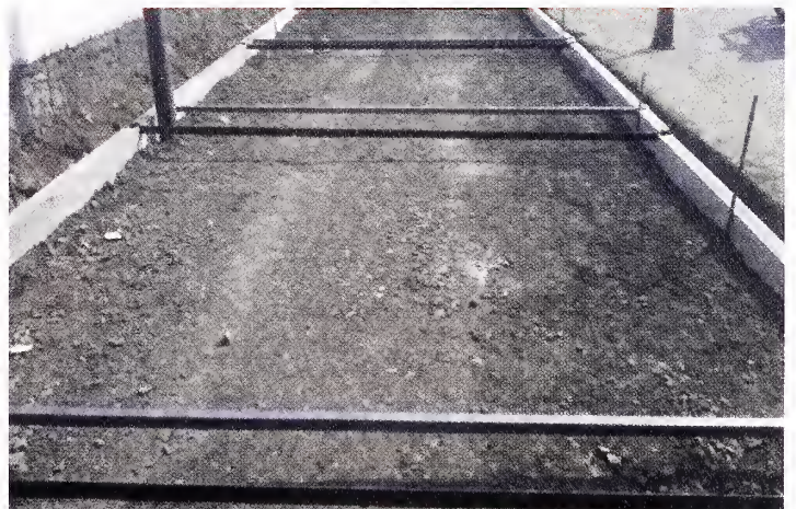
Fig. 5(o) Completed Job-Strips in Stressed Position
