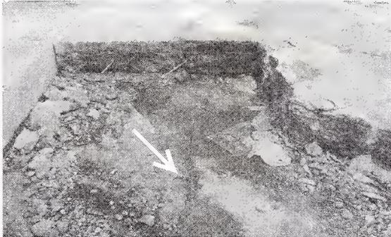
Photo 23) Cracking of DLC Below PQC
