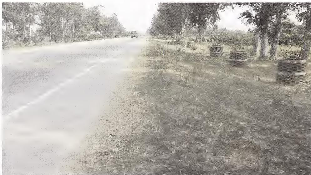
**Photograph 3 - Turfing on Shoulder and Side Slope**
