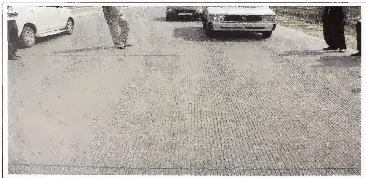
**Fig. 8.7. Abrasion in the Wheel Paths (Longitudinal Tining)**
