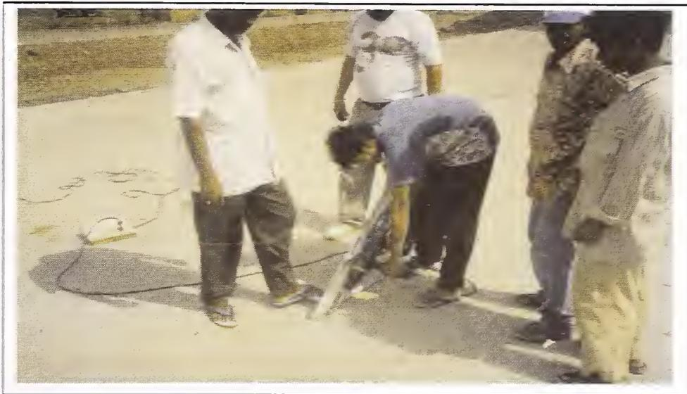
Fig. 7.2. Drilling the Inclined Holes with Angle Template
