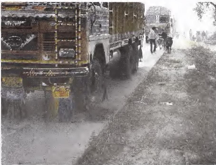
**Photograph 1 - Erosion, Wear and Tear of Soft Earthen Shoulder.
