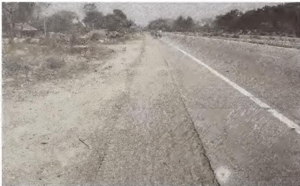
**Photograph 5 - Construction of Brick on Edge (Paved Shoulder)**
