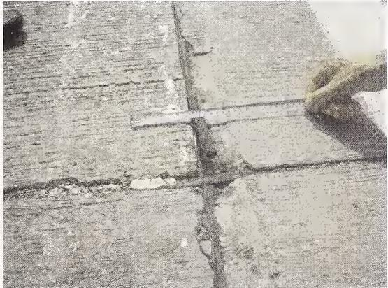
Photo 23) Compressive Seal - Loosening
