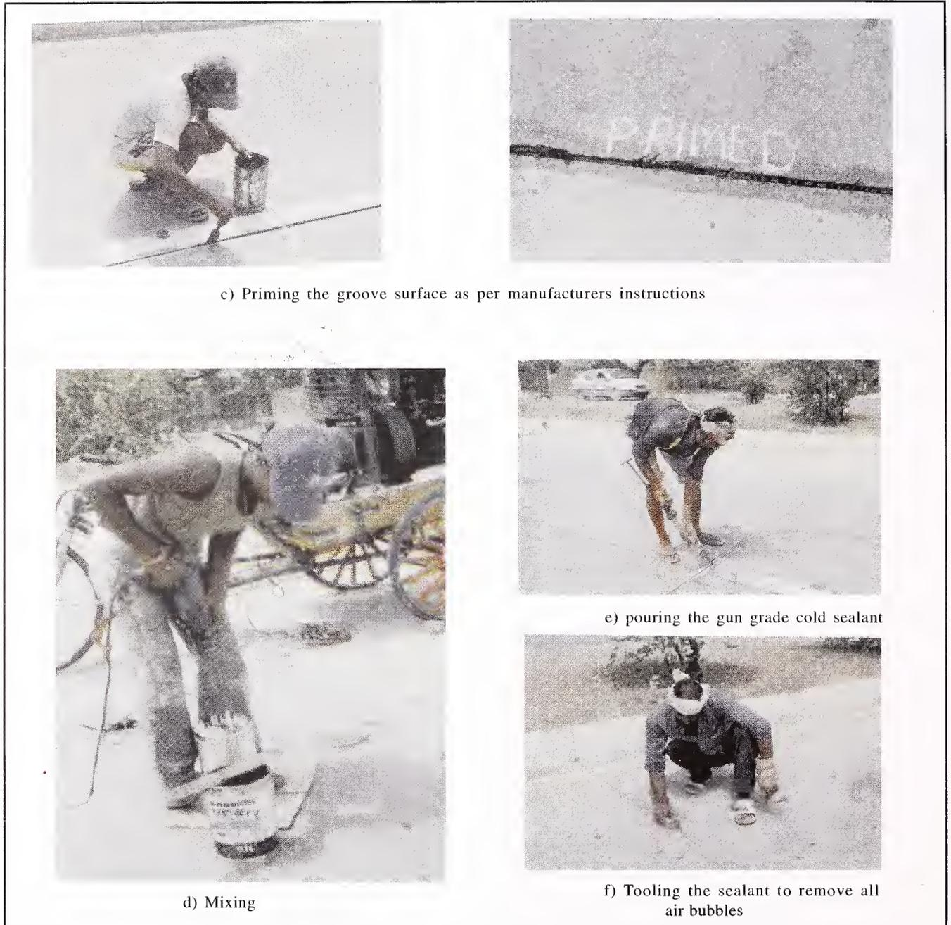
**Fig 6.6. Priming and Reinstallation of PQC Joint Sealant**
