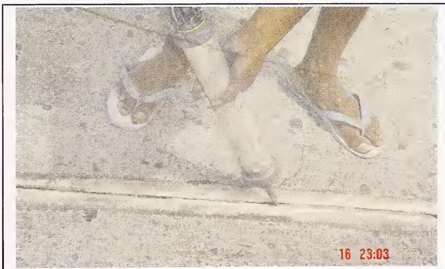
**Fig. 6.2. Joint Resealing**
