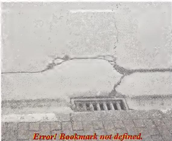
Photo 11) Manhole / Inlet Cracking Failure
