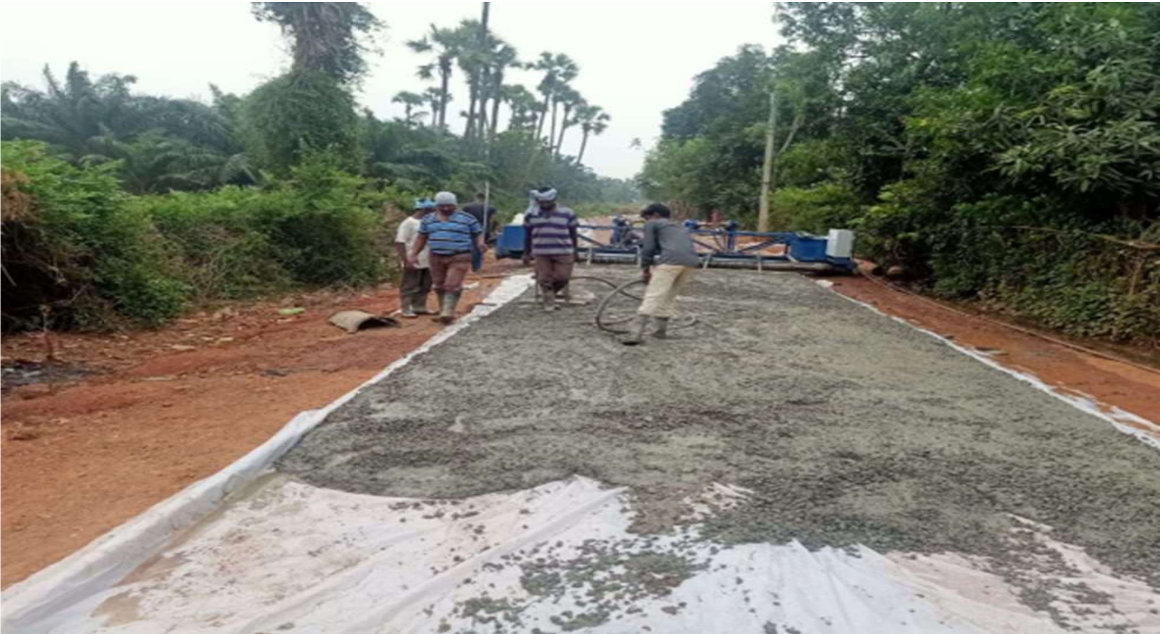
Compaction of Concrete with Needle Vibrator
