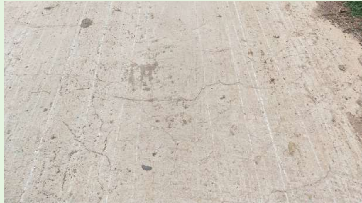
Shrinkage Cracks in CC Pavement
