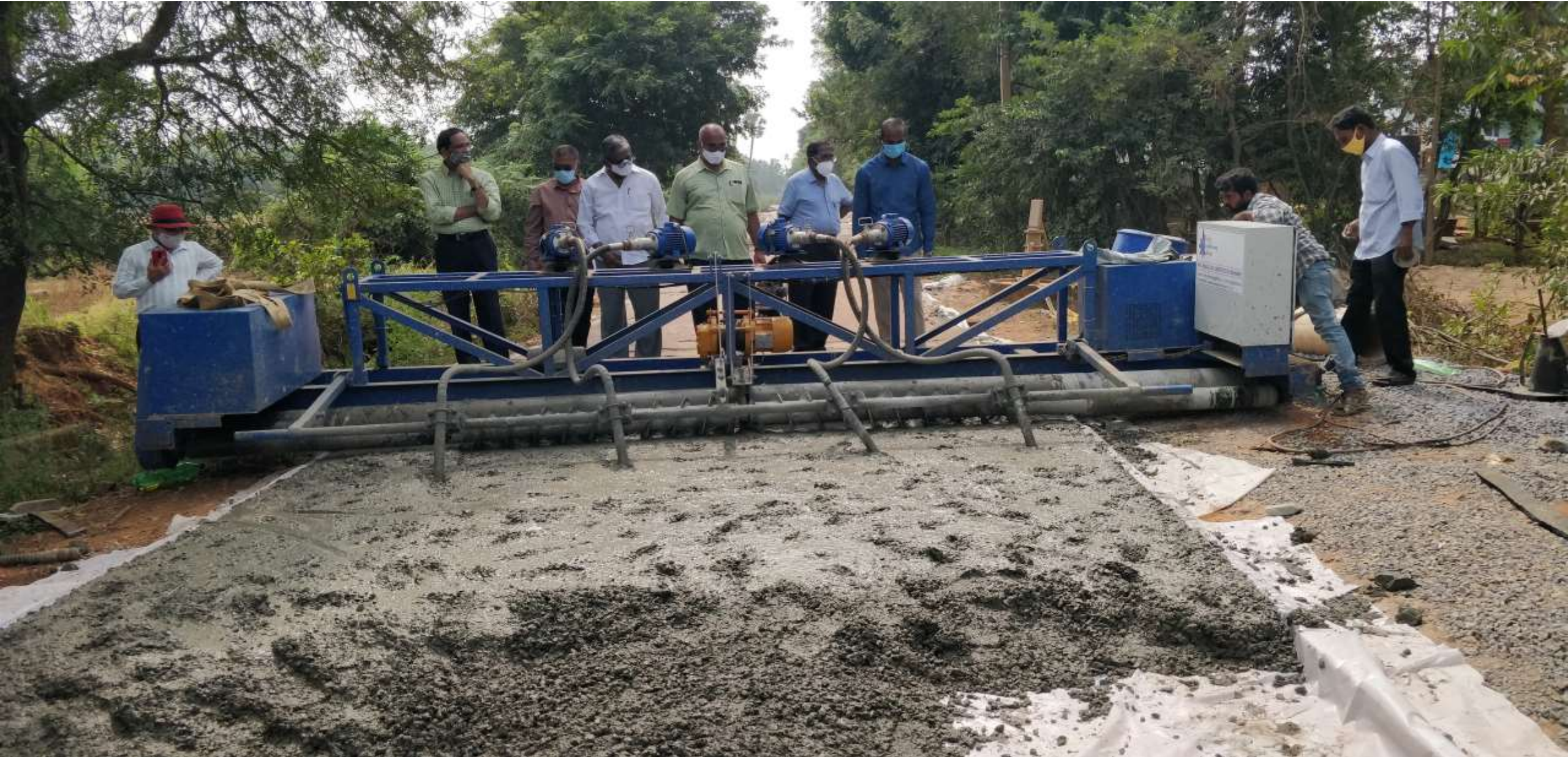
Concrete levelling and compaction with needle vibrators attached to the Screeding machine
