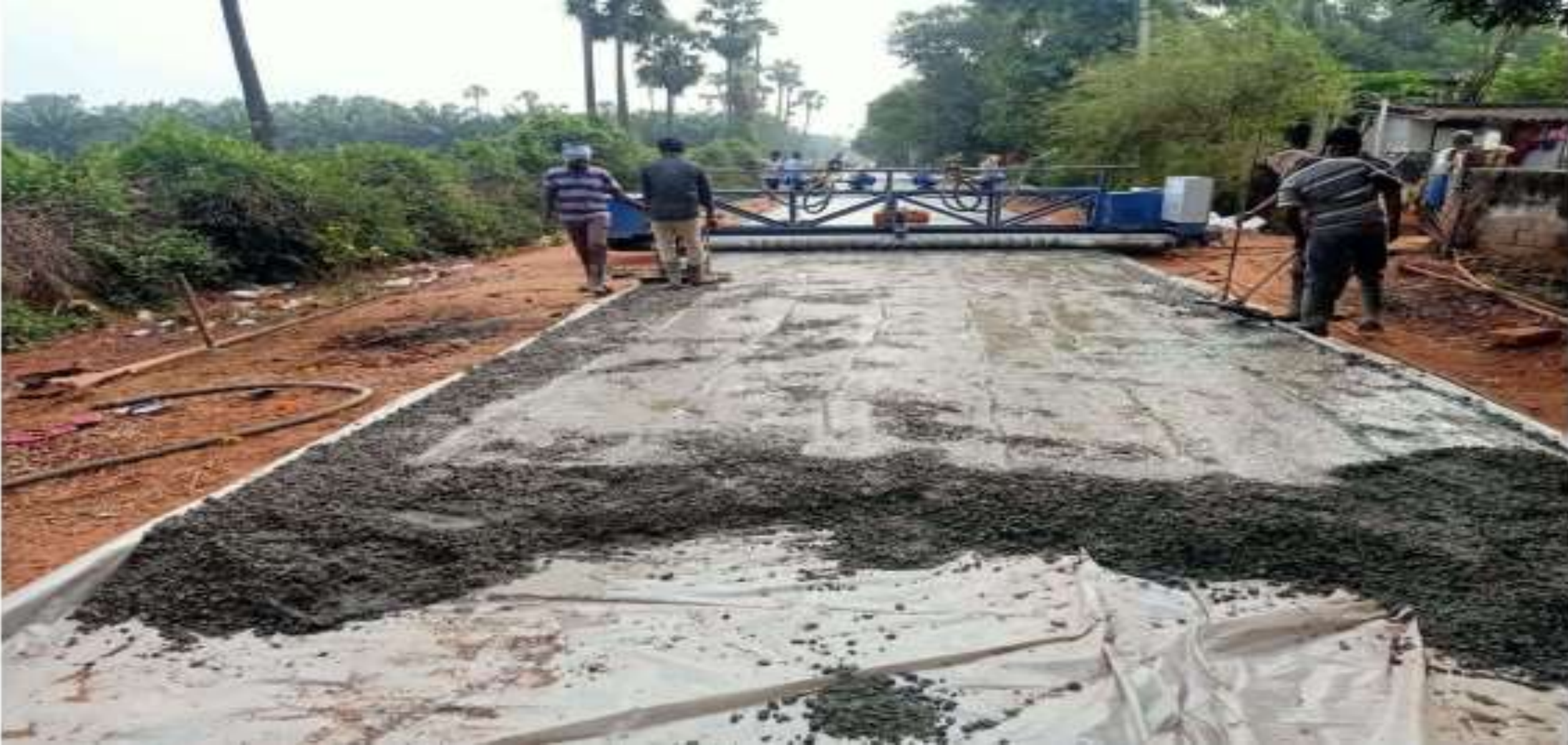
M40 Concrete Laying and levelling with Screeding machine
