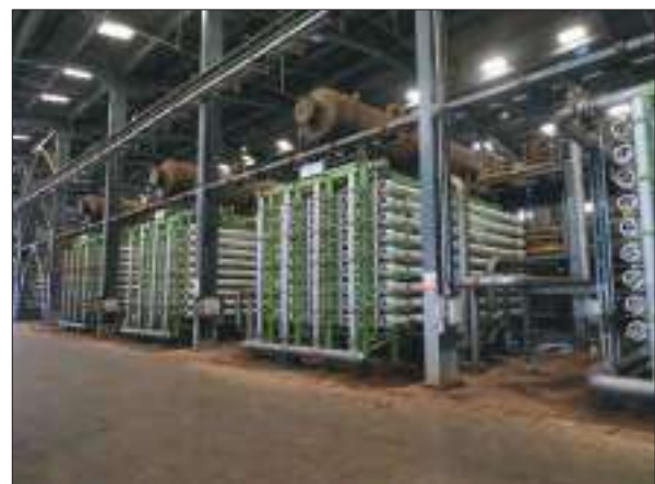
Figure 10.22: RO Membranes Skids
