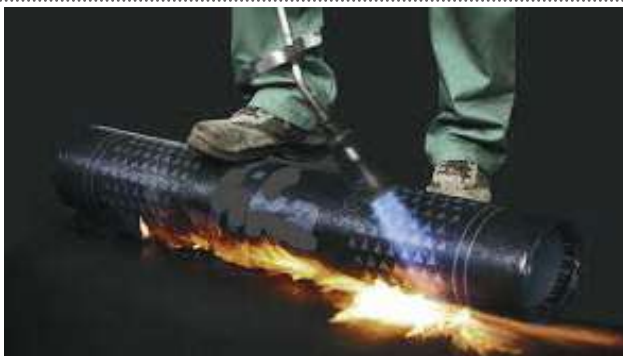
Figure 11.8: Torch application for bituminous wrap coating
