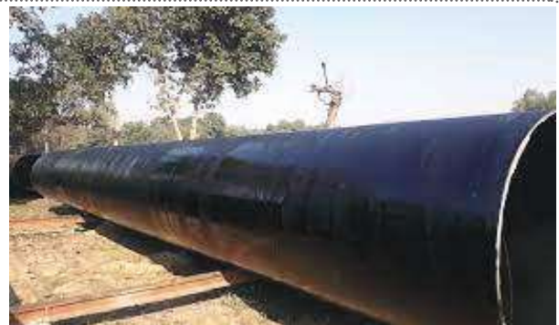
Figure 11.9: Application of tape coating in pipeline
