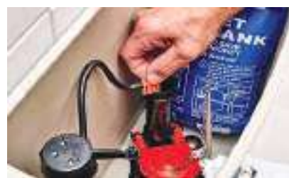
Figure 15.4: Tank bank to save on Toilet flushing
