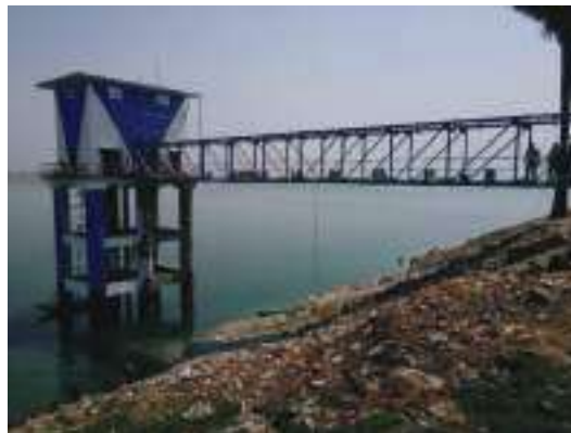
Figure 4.7: Fixed Jetty Intake
