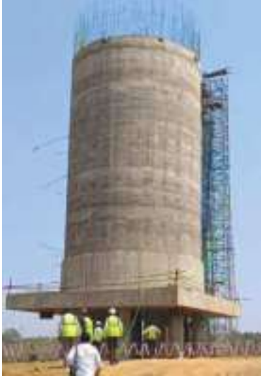
Figure 6.19: 23 m high BPT nearing Completion
