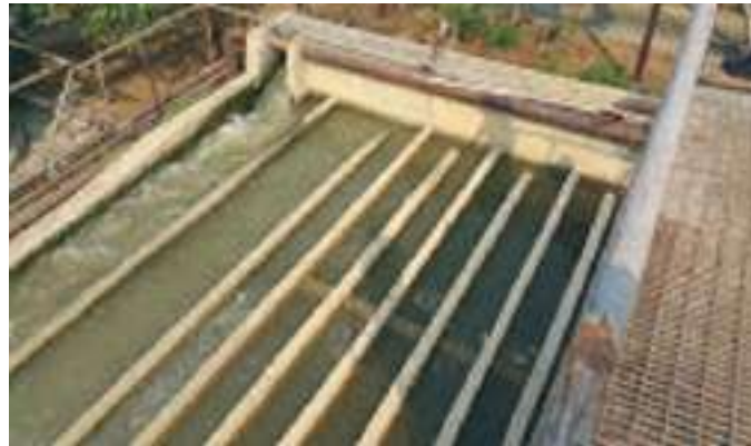
Figure 8.9: Horizontal Flow Baffled Flocculator
