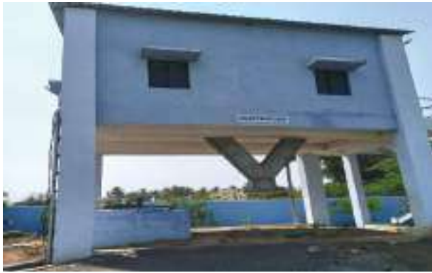
Figure 8.50: Centrifuge Building with "Chute"
