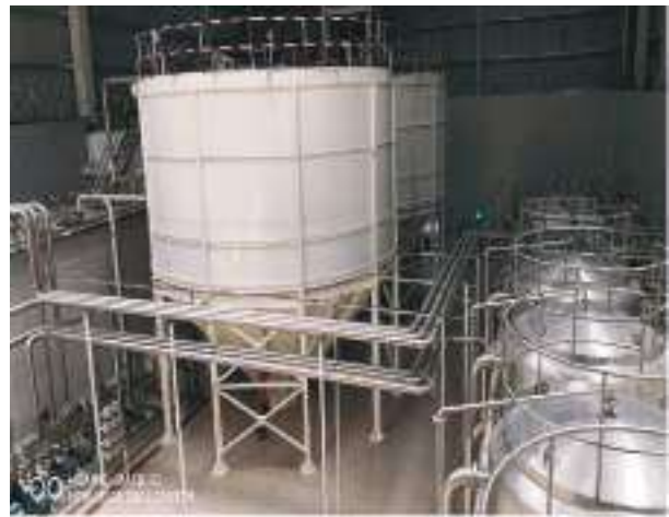
Figure 8.15: Sludge Blanket Clarifier
