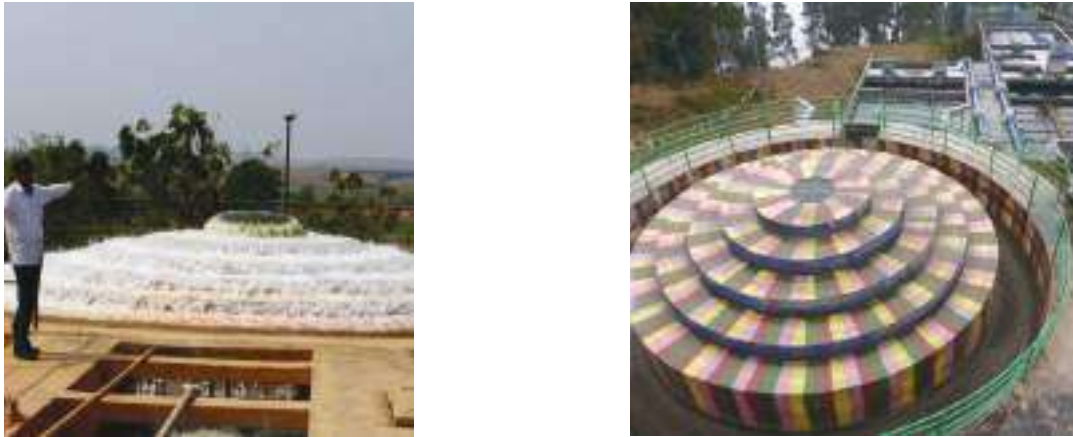
Figure 8.1: Cascade Aerators with Four to Six Steps
