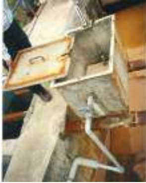
Figure 8.6: Gravity Orifice & Taper valve Dosing Box
