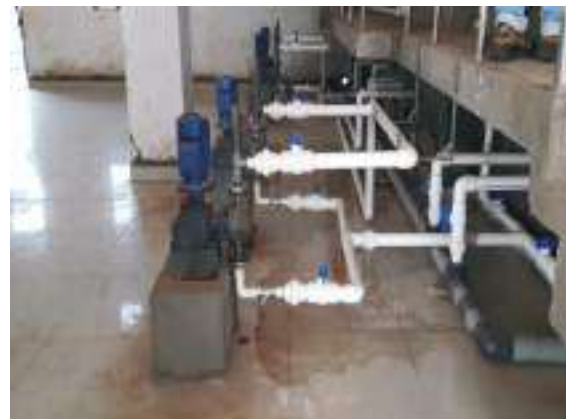
Figure 8.8: Reciprocating / Positive Displacement Pump Chemical Feeders
