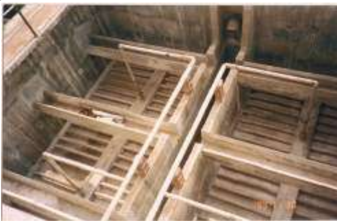
Figure 8.33: Manifold-Laterals Assembly
