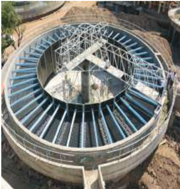
Figure 8.24: Clarissetler with Rotating Scrapper Bridge
