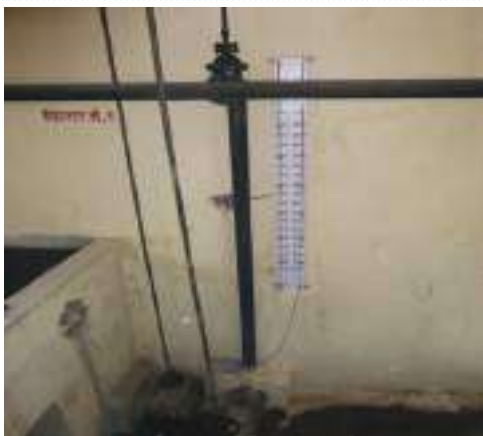
Figure 8.36: Head Loss Indicator (Manometer)
