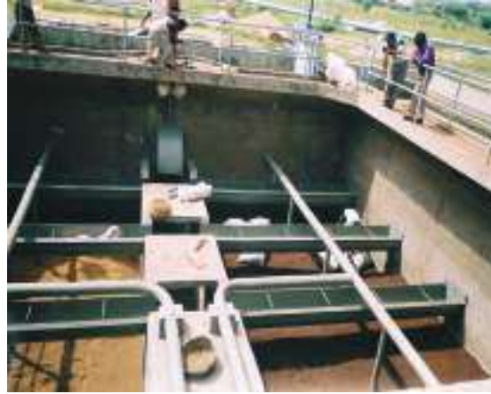
Figure 8.40: Dual Media Filter Bed during Internal Erection and Media Loading
