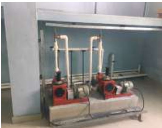
Figure 8.8: Reciprocating / Positive Displacement Pump Chemical Feeders
