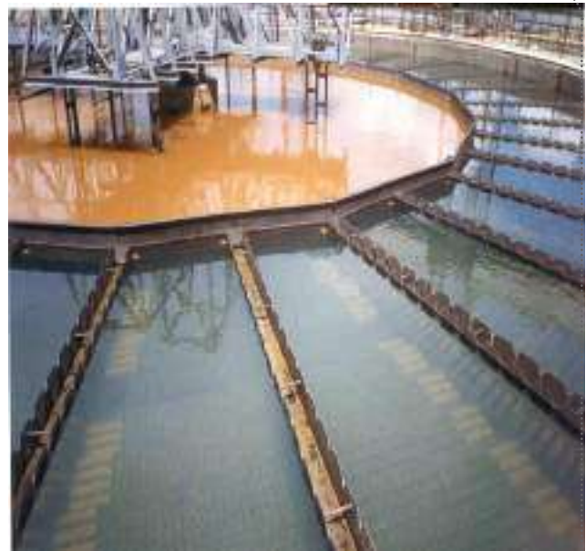
Figure 8.25: Clarissetler with Central Rake
