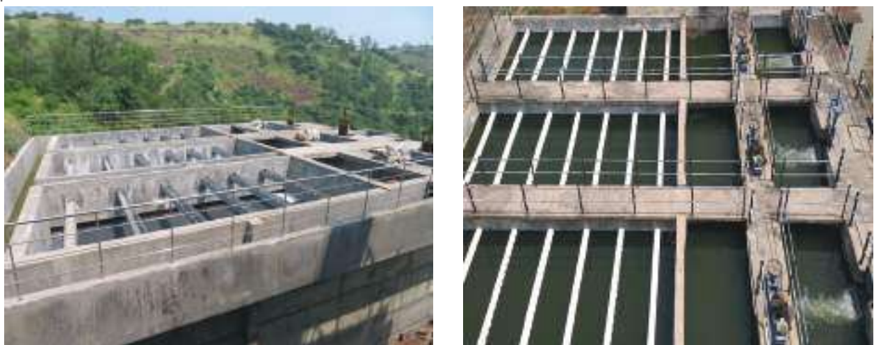
Figure 8.21: Tube Settling and Flocculation under operation Modules & Troughs
