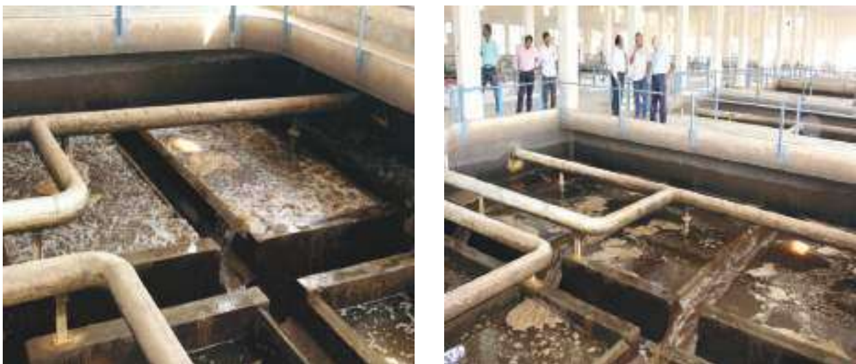
Figure 8.35: Cross-Troughs and Central gutter
