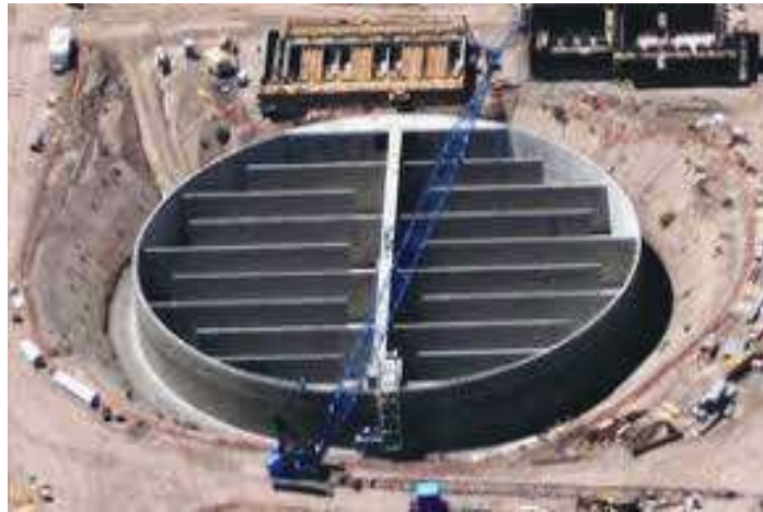
Figure 9.13: Circular contact tank under construction
