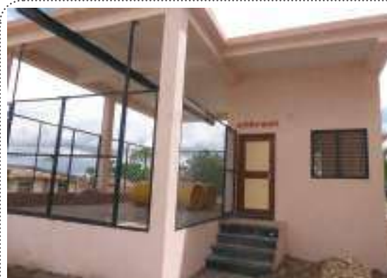
Figure 9.8: Chlorination Room and tonner yard at Ghulewadi (10 MLD) WTP, Dist. Ahemadnagar, Maharashtra
