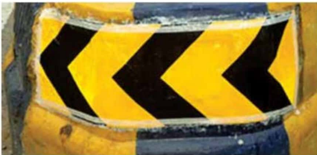
Fig. 7.15. Typical Illustration of Placement of Flexible Object Markers
