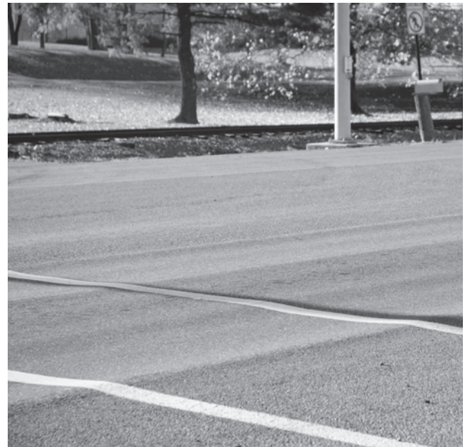
FIGURE 10.1 Rutting Shown at an Intersection
