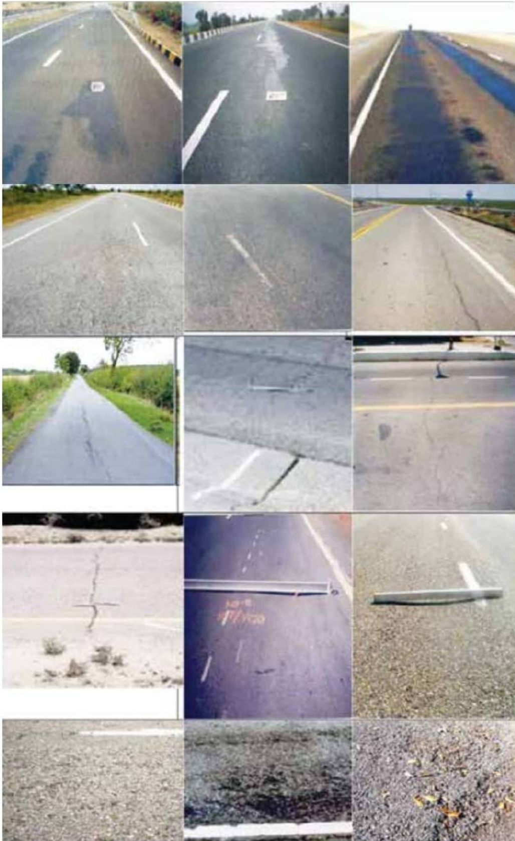
Annexe 12.1. Photographs of Distress on Flexible Pavements
