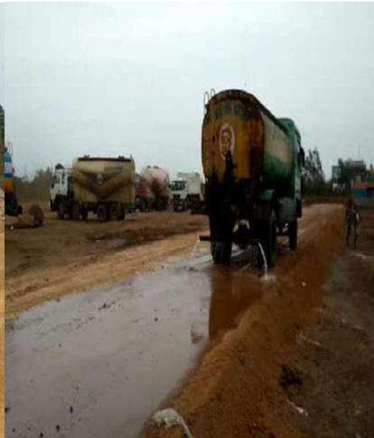
Fig 8. Curing of finished Stabilized layer.
