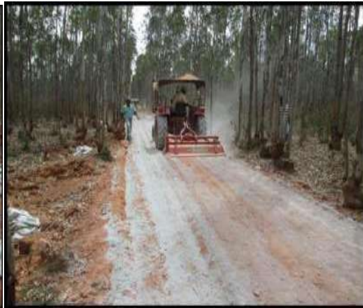
Fig 4. View of Dry mixing with Rotavator
