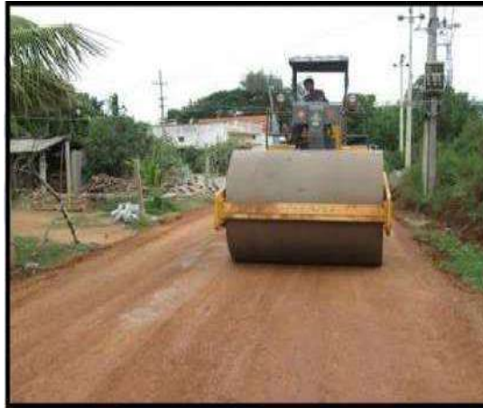
Fig 7. View of rolling after Grading
