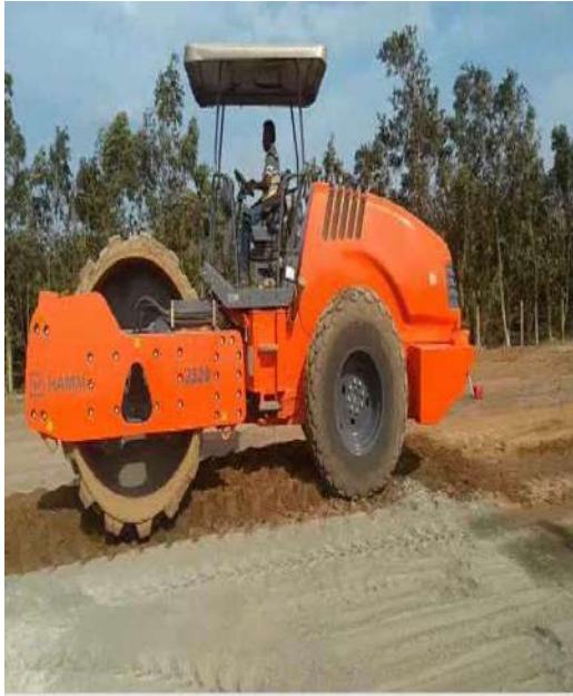
Fig 5. Rolling with 20T Pad foot Roller
