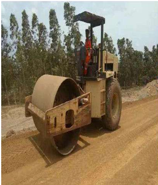
Fig 7. Rolling with Vibratory Roller
