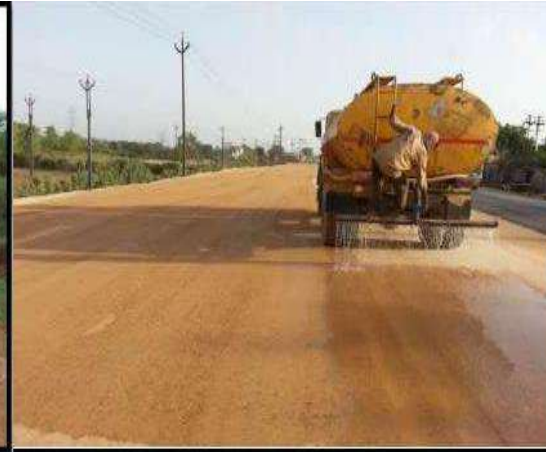
Fig 8. View of curing of finished Stabilized layer
