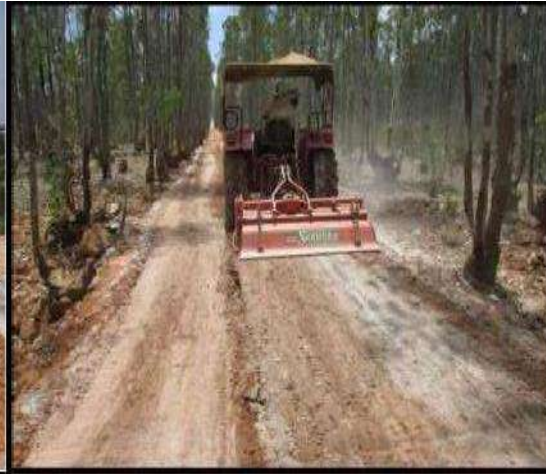
Fig6. View of Wet Mixing by Rotavator
