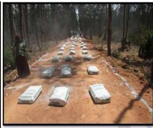
Fig 2. View of Cement bags laying for Stabilized Layer.
