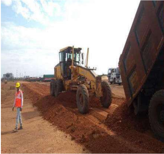
Fig 1. Spreading of construction material For stabilized layer
