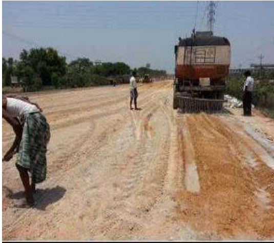
Fig5. View of Water Addition
