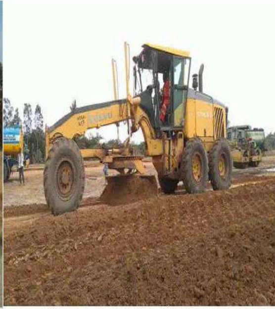
Fig 6. Grading with Grader
