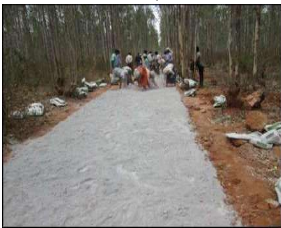
Fig 3. View of Cement Spreading
