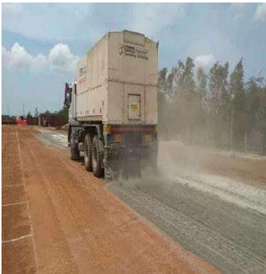
Fig 3. High End Cement Sreader
