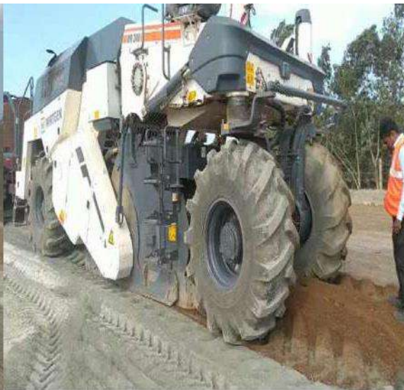
Fig 4. Mixing with Recycler at OMC
