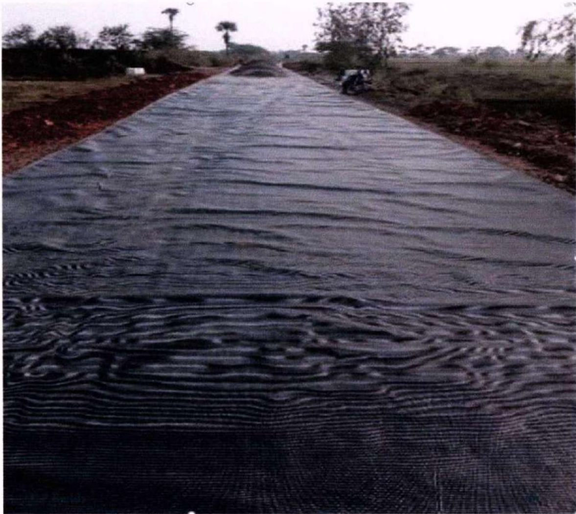
Photograph showing the process of laying PP Woven Geotextile and back dumping of GSB material is in progress.
