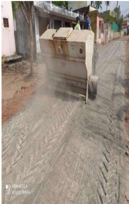
Additive Spreading
