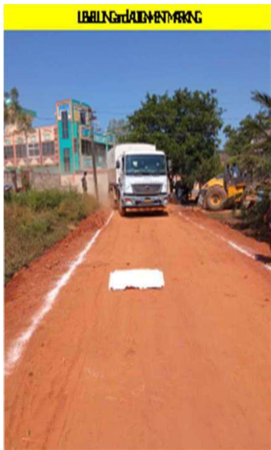
Levelling with barrowed soil and lime marking
