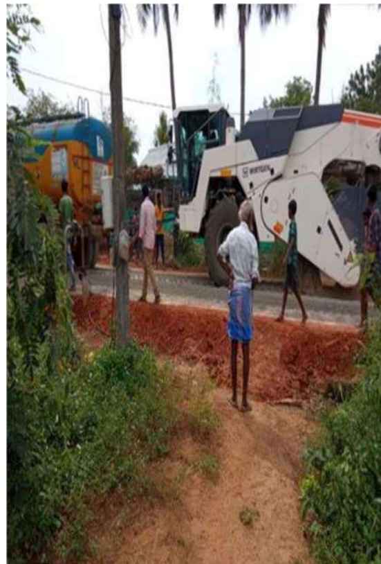
Recycler attached with Water Tanker
