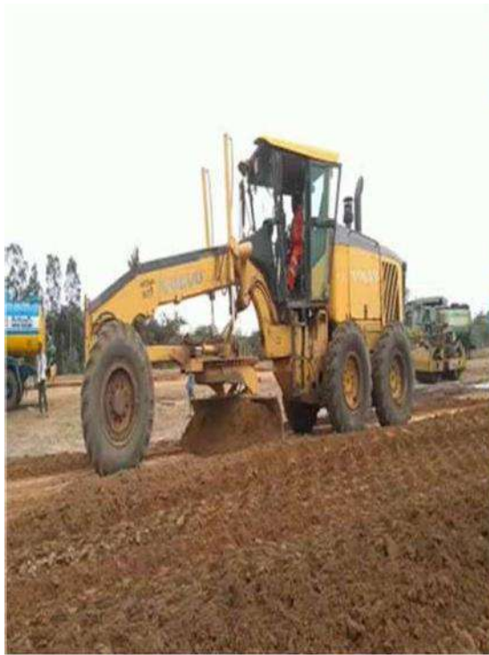
Grading with Motor Grader
