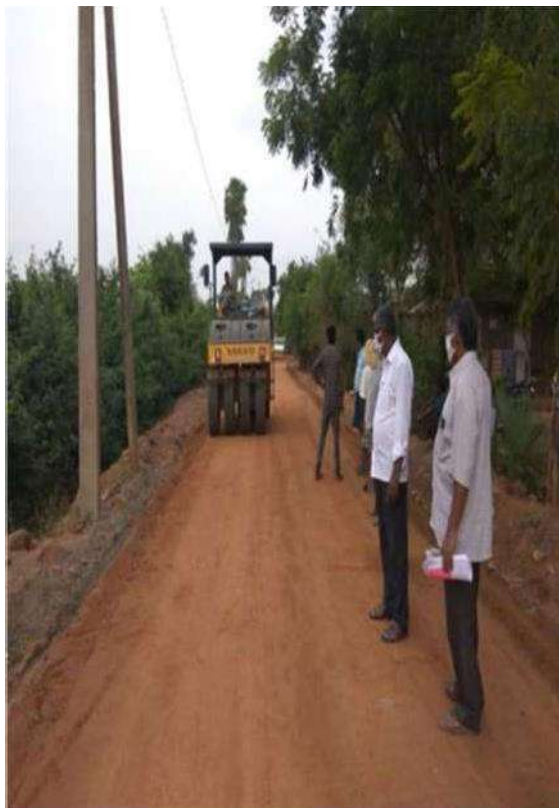
Rolling with PTM Roller to get Smooth Surface
