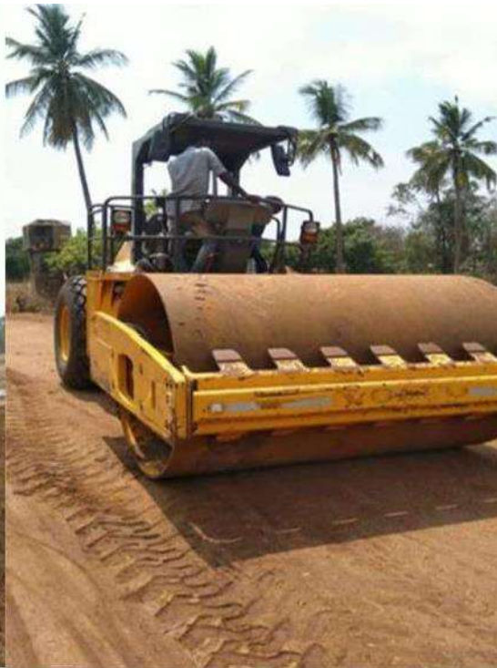
Plain Rolling with Vibratory Roller
