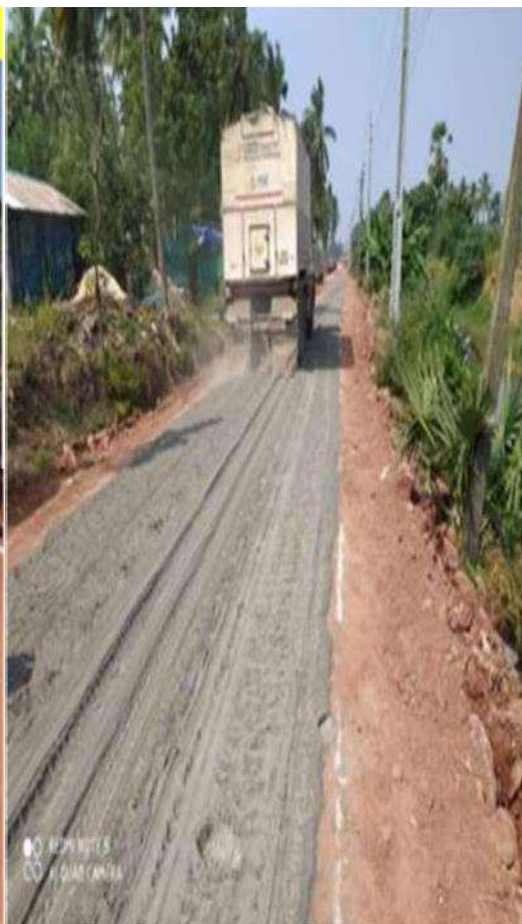
Cement Spreading with Cement Spreader
