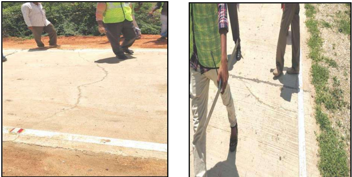
Fig1. Cracks observed in APRRP CC roads
