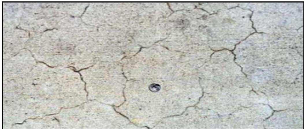
Fig 4. Cracking cracks in CC Pavements
