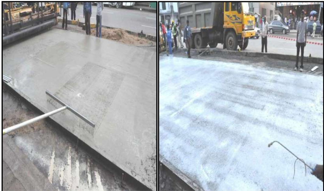
Fig 10. Texturing and Intermediate Curing with Application of Curing Compound
