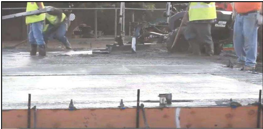
Fig 8. Slab is ready for Initial Curing
