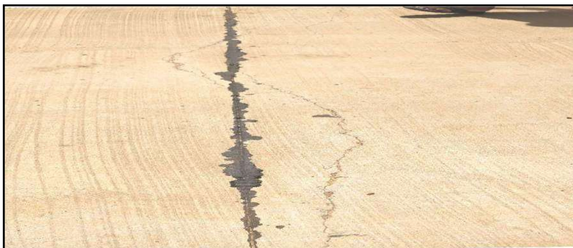
Fig 12. Cracks due to late sawing of Initial cut of CC road
