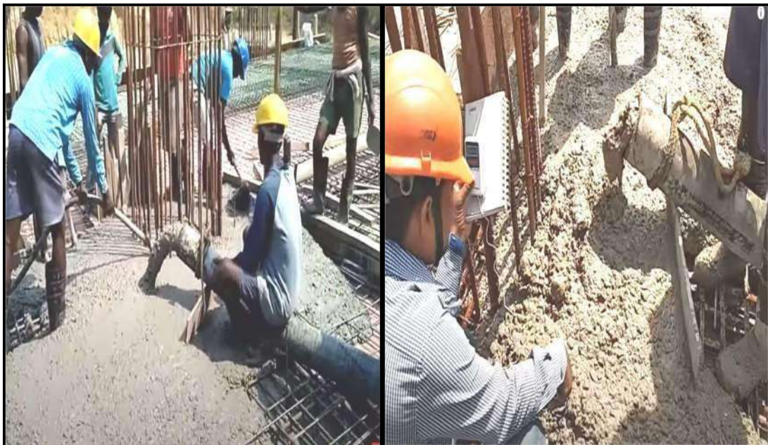
Fig 7. EXCESS WATER in THE MIX (Wrong Method of placing concrete)
