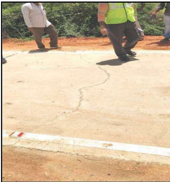
Fig1. Cracks observed in APRRP CC roads
