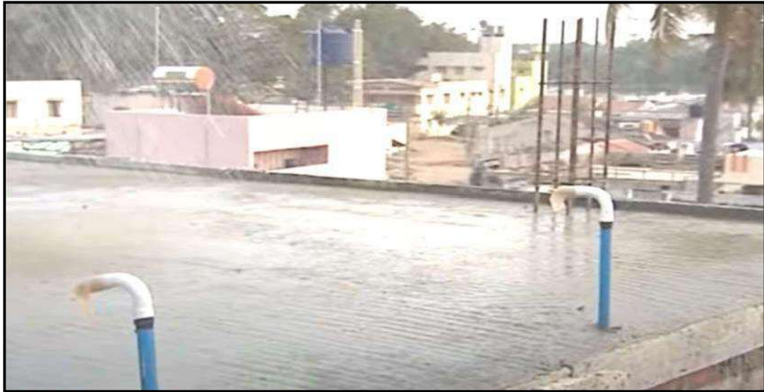
Fig 9. Initial Curing with Sprinkling of Water
