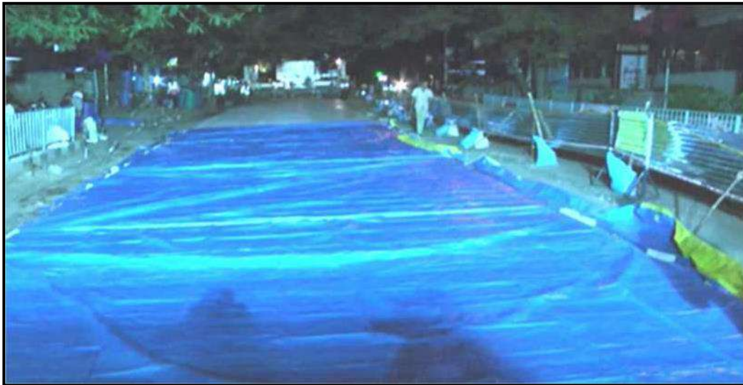
Fig 5. Concrete slabs covered by Plastic sheet
