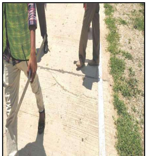
Fig1. Cracks observed in APRRP CC roads
