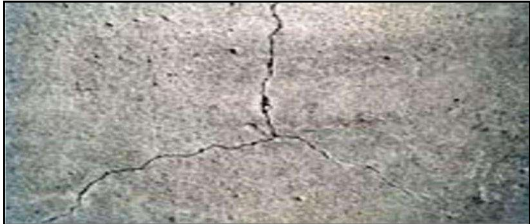
Fig 3. Drying shrinkage cracks in CC pavement
