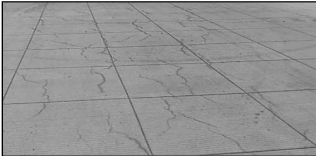
Fig 2. Plastic shrinkage cracks in CC pavement
