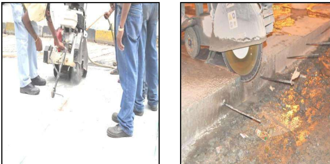
Fig 11. Sawing Depth H/3 to H/4
