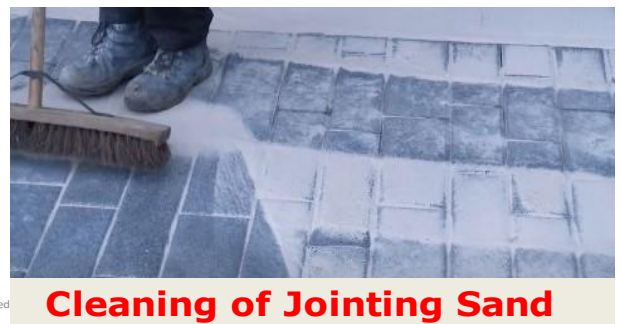
Sweeping in the Jointing Sand
