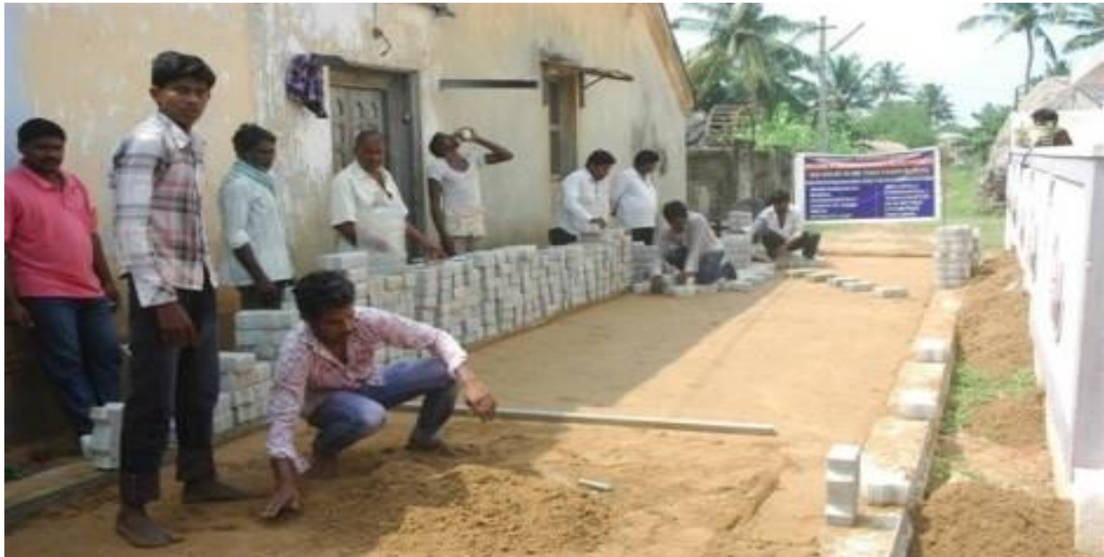
Precast M40 concrete blocks of 80mm thick laying in progress after sectioning the sand bed.
