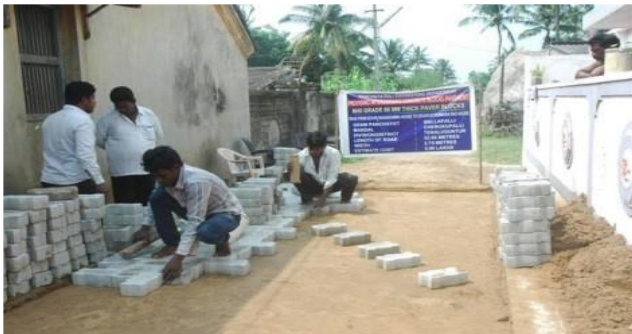
Precast M40 concrete blocks of 80mm thick : Laying in Progress
